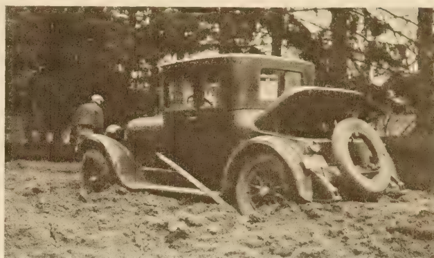
FIGURE 63.—TYPICAL FROST BOIL CAUSED BY LACK OF STABILITY IN SOIL
